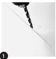
Check product orientation. Mark hole positions from brackets pre installed on MOMO Sauna base (2 per metre/40") and drill if required.
